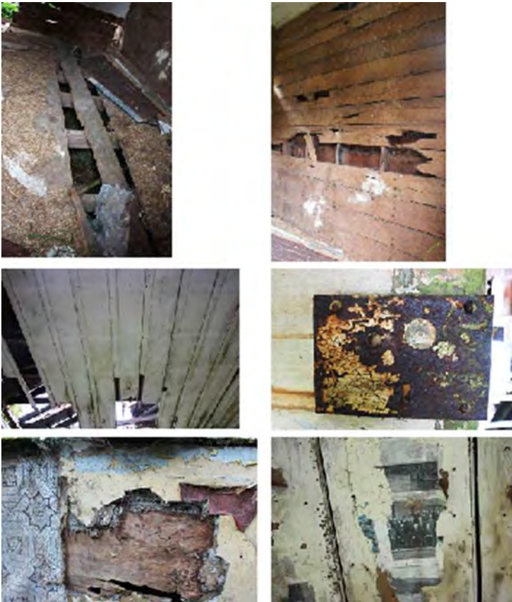
Figure 82 – Woodthorpe interior. Top (left) area of surviving floor covered in straw and (right) surviving wood lining; Middle (left) remnant board and batten ceiling and (right) Carpenters lock; Bottom (left) wall coverings in former kitchen area and (right) newspaper cuttings lining the lean-to ceiling
