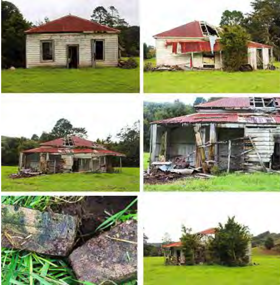
Figure 80 – Woodthorpe exterior. Top (left) looking W front elevation and (right) looking S at verandah on north elevation; Middle (left) looking E at lean-to and (right) looking E at N end of lean-to ; Bottom (left) wire cut bricks from the original chimney now gone and (right) looking N at southern elevation
