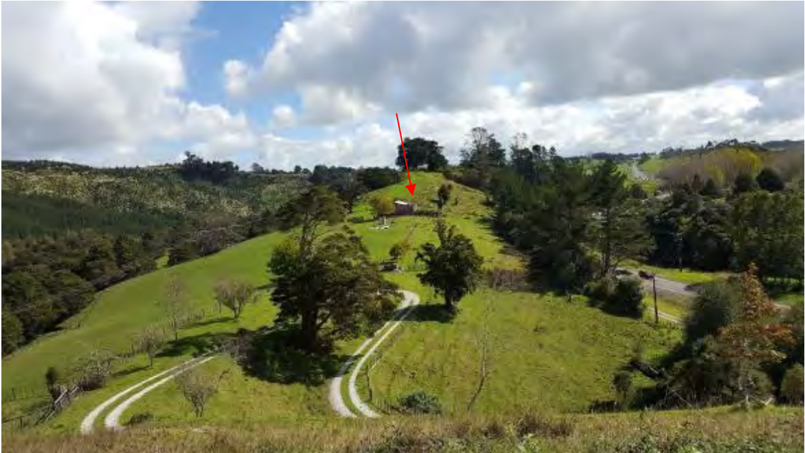
Figure 66 – Location of the woolshed at 1207 SH1, facing north
